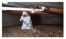
**4.** Seal up all areas where outside air could enter the crawl space such as vents and pipe penetrations around the perimeter. This can be done using our spray foam insulation kits, can foam, or caulking.
