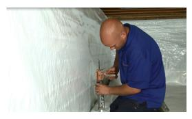
**7c** Tape all seams and around piers using the seam tape. NOTE: Try to get the liner and tape to be parallel to the ground. This is purely cosmetic, but makes for a cleaner finish.
